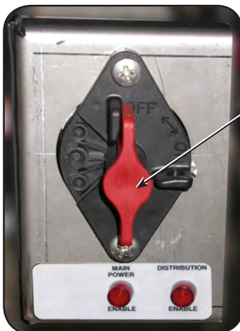
BATTERY DISCONNECT SWITCH
